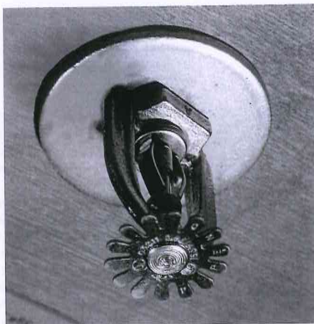
D-1.5: sprinklerkop
